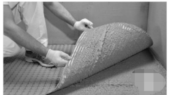
align it with the previous one without overlapping. Align the square reliefs to facilitate the installation of the heating cables.
